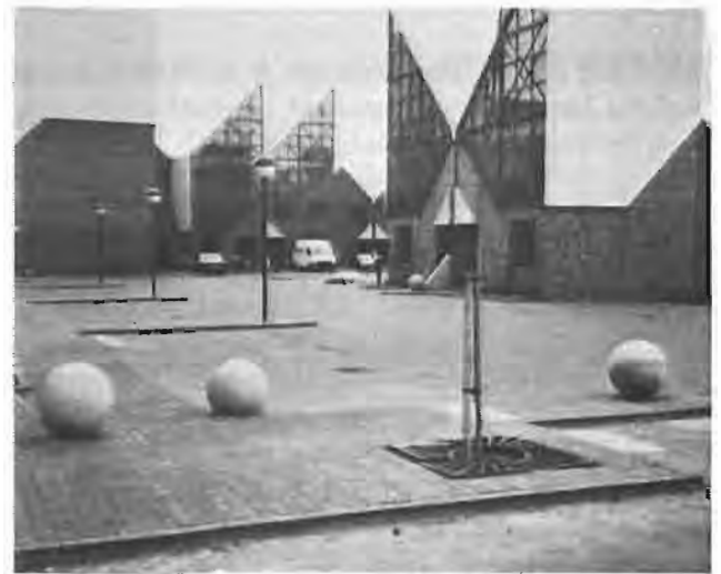
FIGURE 4-1. Roofs and pavement leave little habitat for wildlife.
